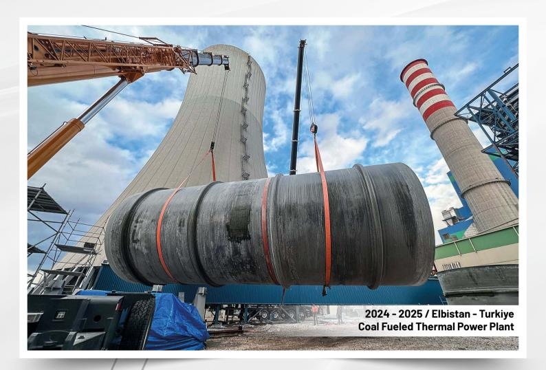
Site fabricated GRP pipeline Thermal power plant chimney line 8100 mm outer diameter & 130 meter lenght
