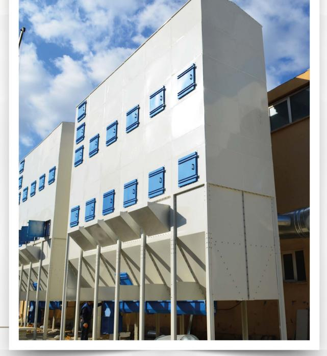
Dust particles emerging during the production process of furniture, chipboard, woodworking and sawmills are seperated from the work environment thanks to modular filter systems. The sucked ambient air is cleaned by a modular bag filter and returned to the factory to prevent negative pressure and excessive heat loss.
